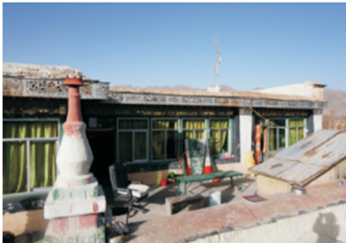
图 1 典型建筑 Fig.1 Typical building
