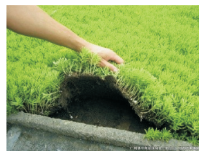
图4 卷铺式佛甲草绿化屋面施工流程及实景 Fig.4 Construction process and real scene of rolling flooring floss grass green roof
