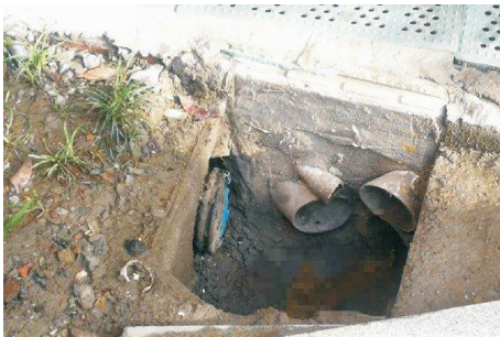
图6 排水管道混接错接现象 Fig. 6 Mixed connection and wrong connection of drainage pipes
